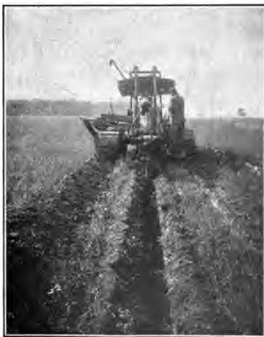
FIG. 200. — Drainage machine at work.
